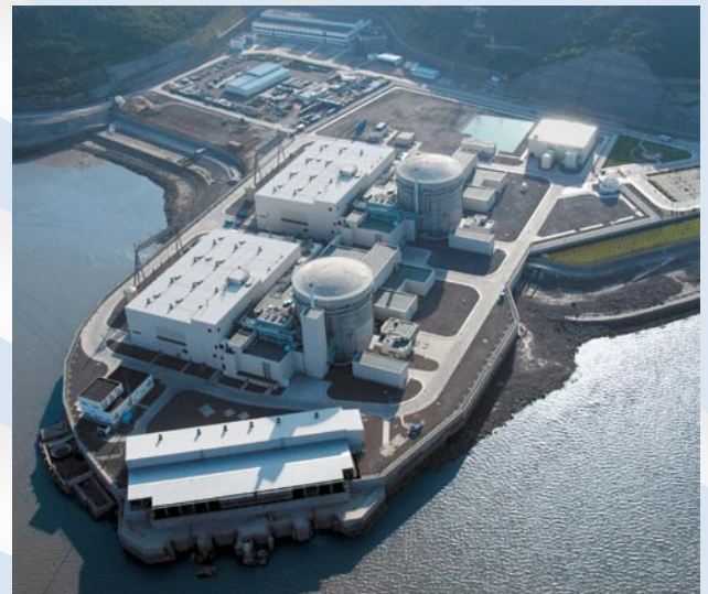
Fig. 1. The Safety Shutdown System 2 (SDS 2), based on proven VME technology, monitors safety critical parameters at the Qinshan Phase III Nuclear Power Station in China.
