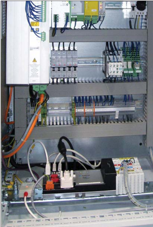
The Kontron ThinkIO-Duo provides standard PC connectivity as well as industrial fieldbus and industrial Ethernet interfaces in a single, ultra-compact unit.
